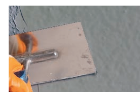
1. PCC-fine mortar Nafufill KM 103 or Nafufill KM 110
